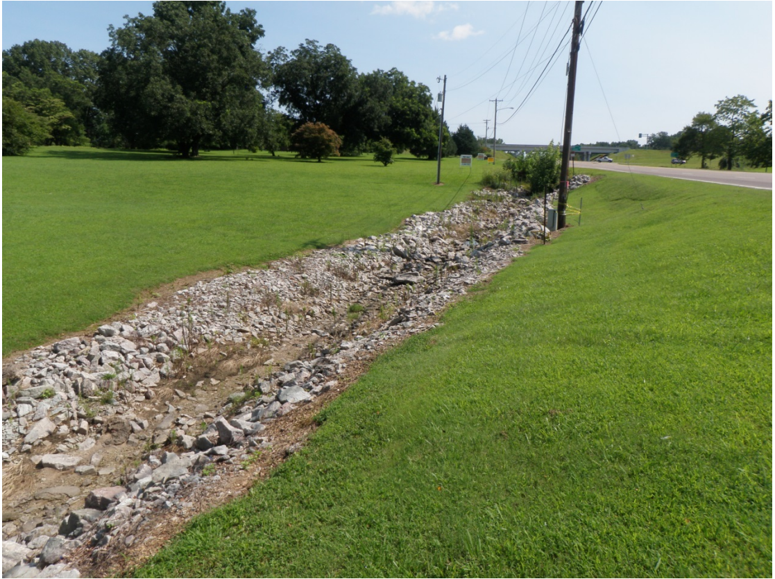
WWC-1 Looking East Towards Intersection
